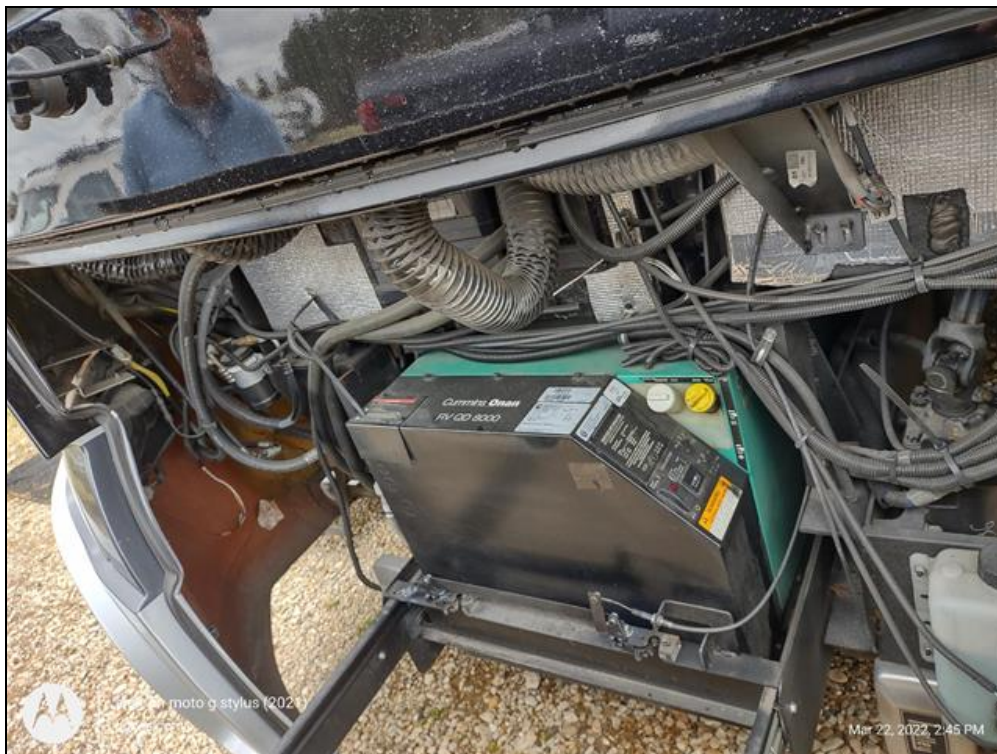
Front mounted Onan 8000 watt Generator
