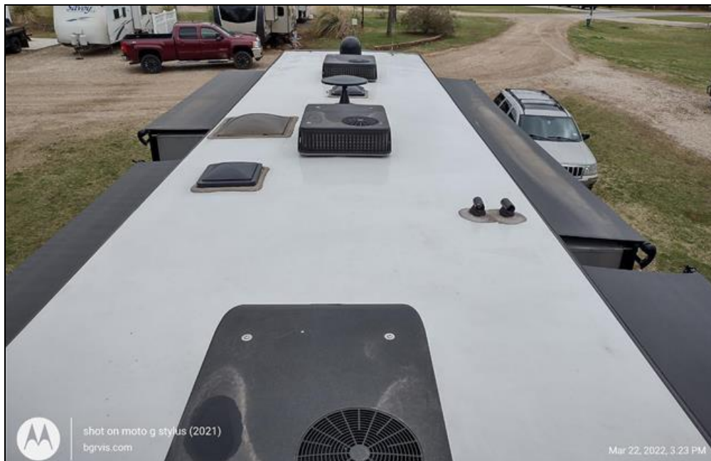
Roof Overview Rear to Back
